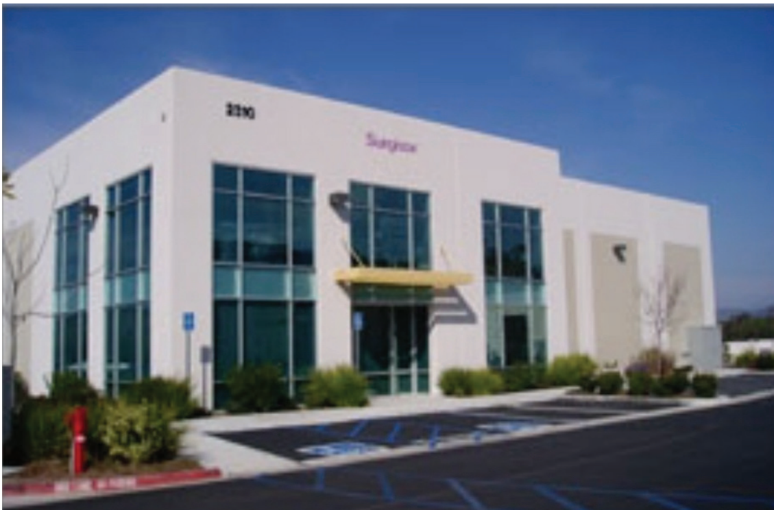
Vista, CA Manufacturing Facility
